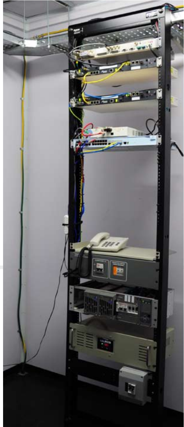
Figura 7: bastidor de equipos dentro del shelter. / Figure 7: equipment rack inside the shelter.
